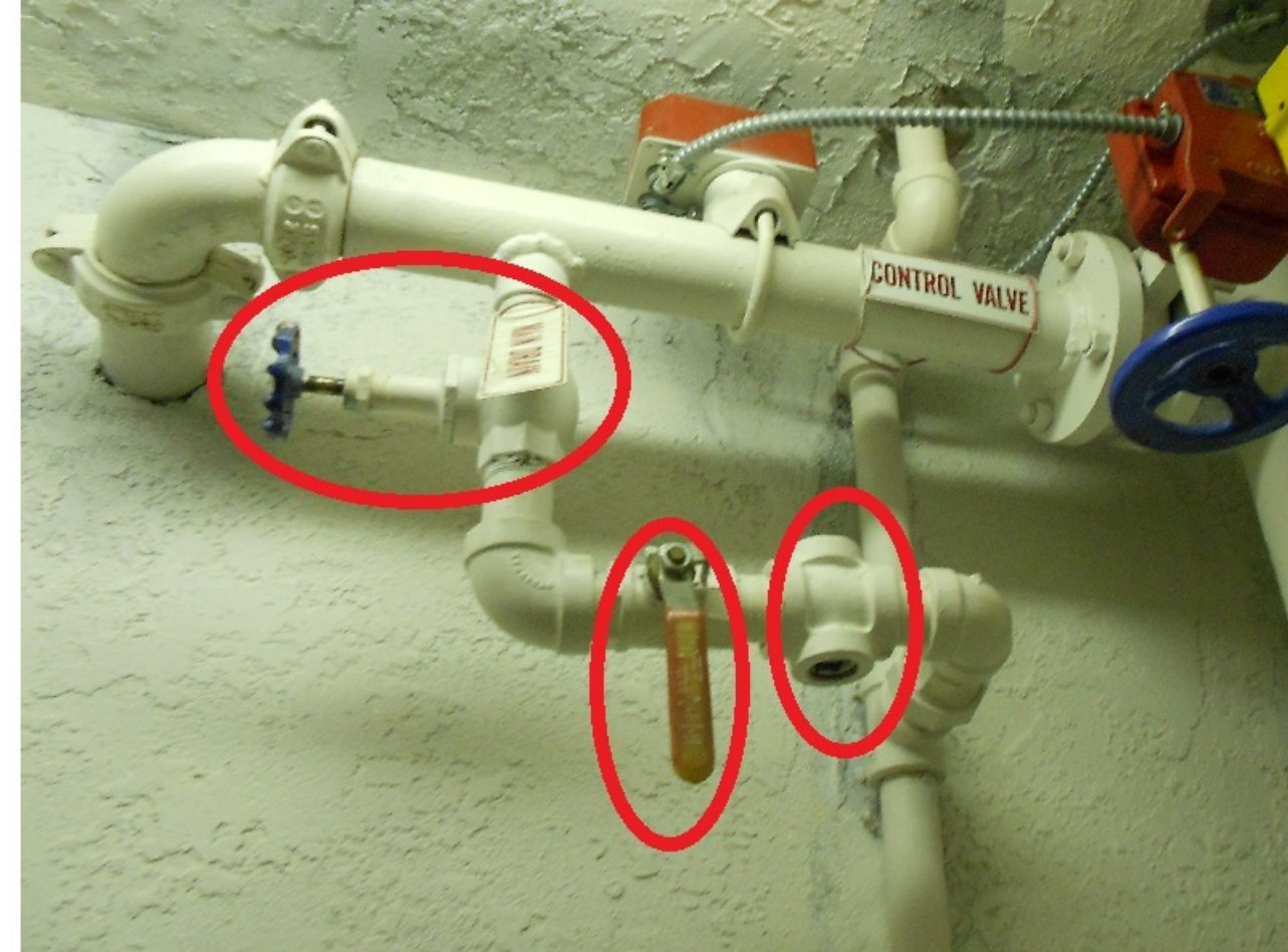
Traditional Valve Set for Fire Sprinkler Inspection
